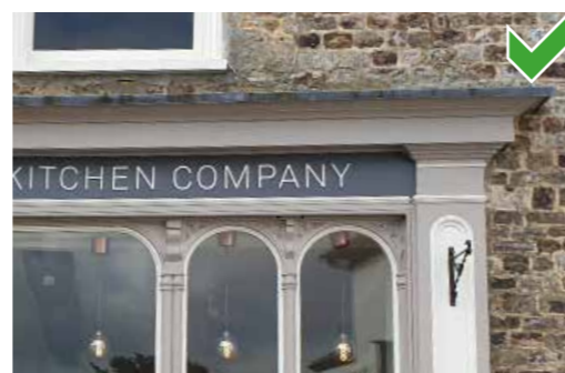
lead covered cornice providing protection for signage below.
